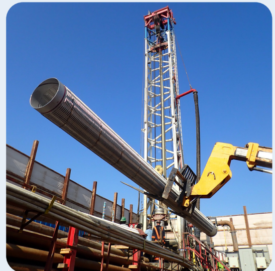
Gage Well Replacement
