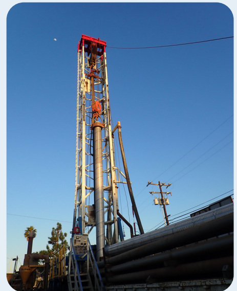
Compton-Doty Well Replacement
