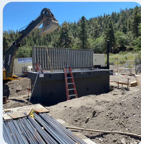
Government Canyon Site Improvement Project
