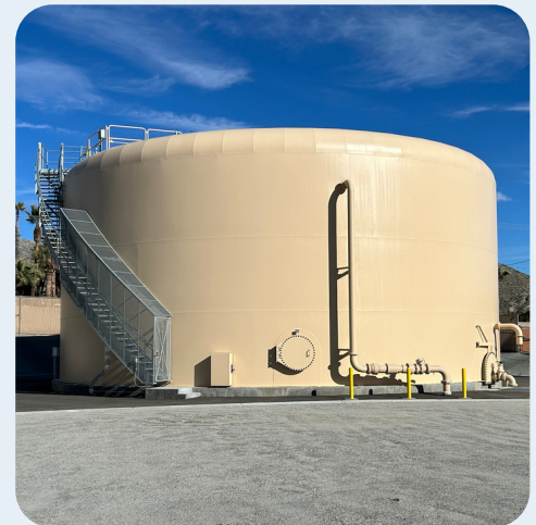
Mojave Booster, Reservoir and Generator Project
