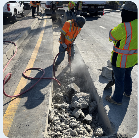
Willow Pass Road Pipeline
