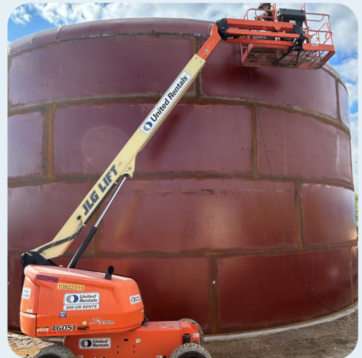
Wayhill Reservoirs Replacement
