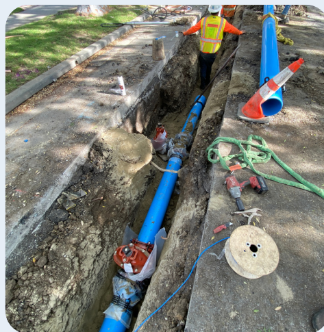
Mentone Main Replacement Project
