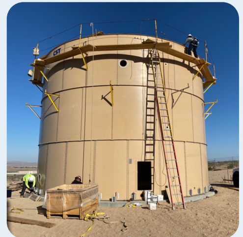
Lenwood Seismic Coupling Project
