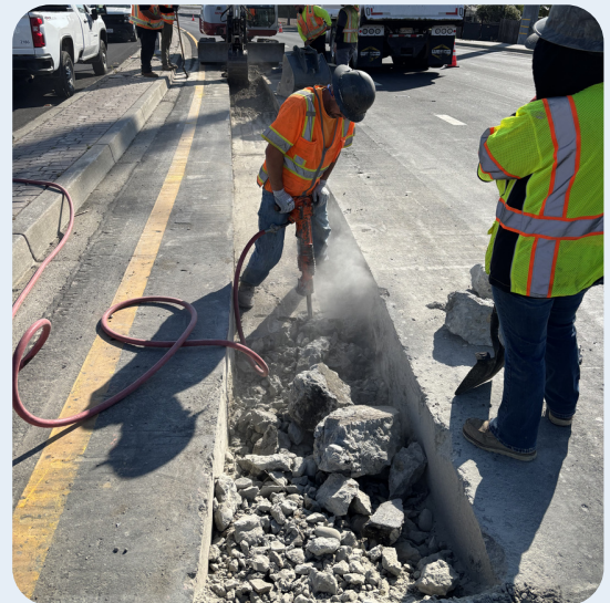
Willow Pass Road Pipeline
