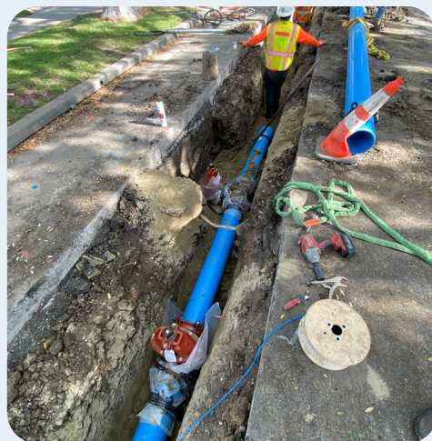
Mentone Main Replacement Project
