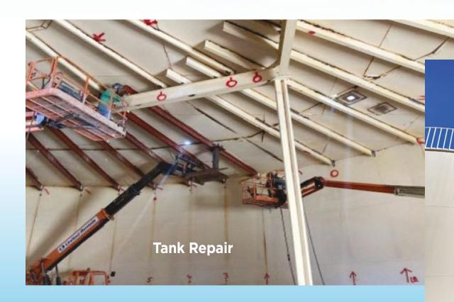
Athens Tank Rafter Repair - Recoat the interior and exterior and upgrade required safety, health, structural, and seismic modification of Athens tank in the Southwest system.
