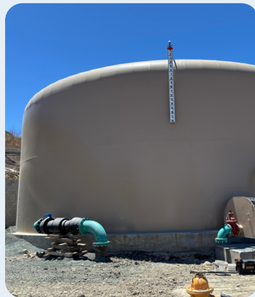
Jack Ranch Reservoir
