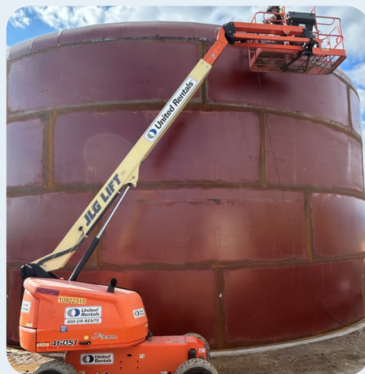
Wayhill Reservoirs Replacement
